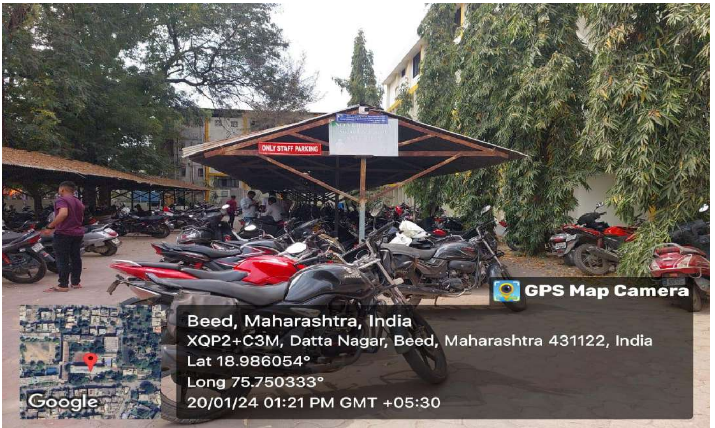
Parking Area Renovated
