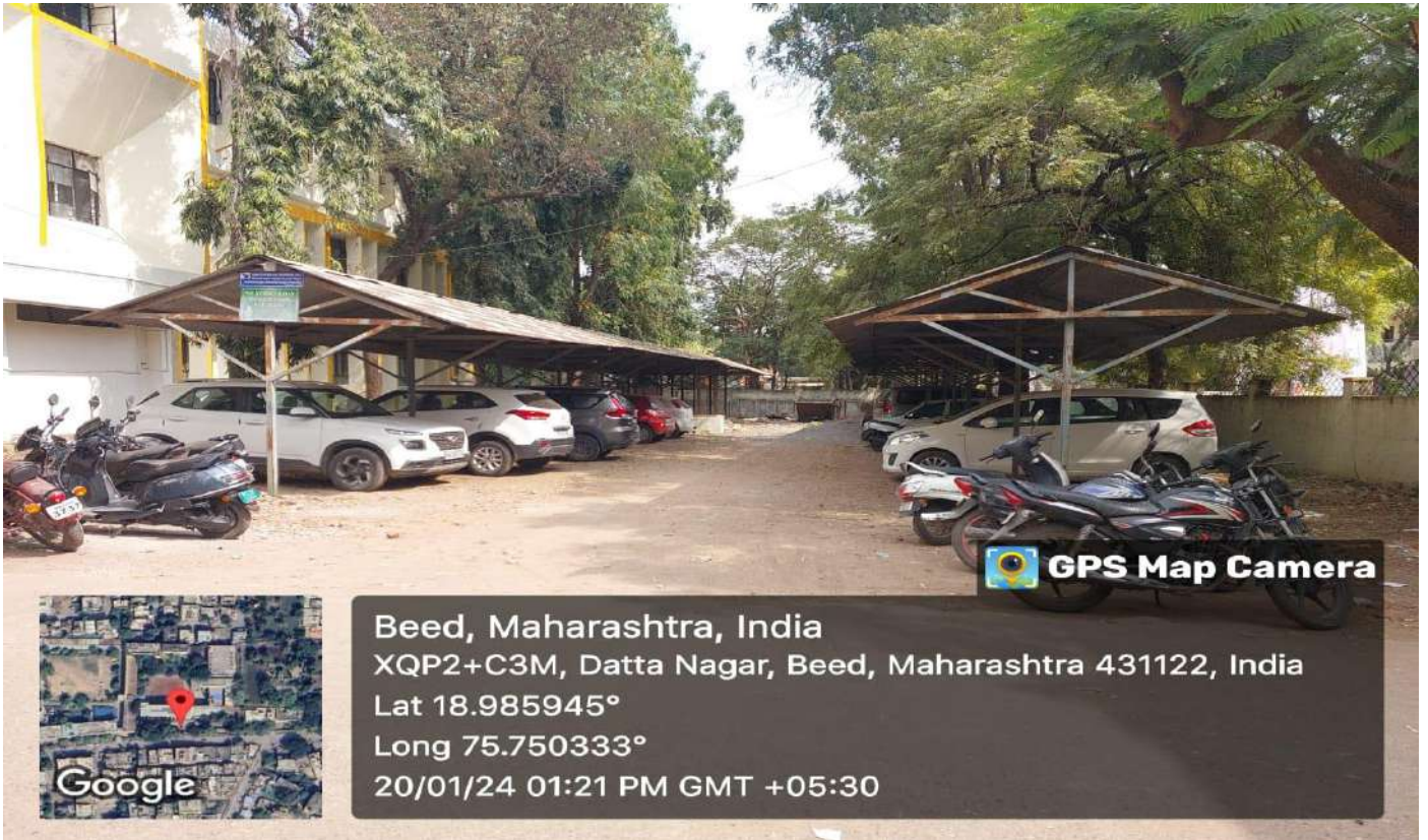
Parking Area Renovated
